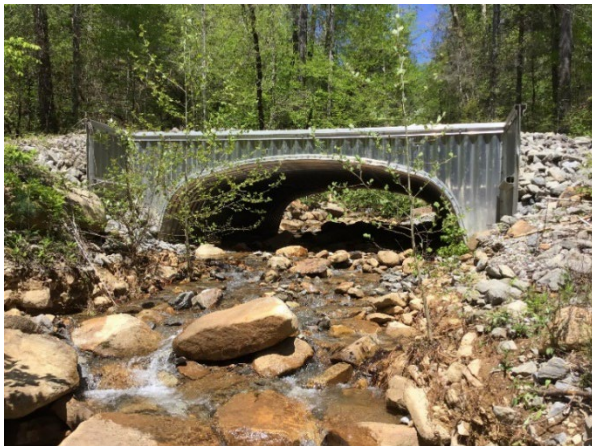
Culvert replacement to improve natural stream flow and aquatic habitat. .
